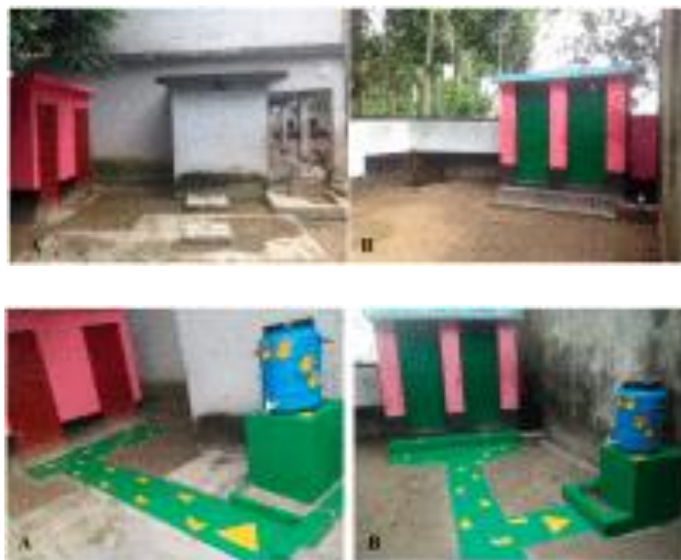
Figure 2.11 School latrine and water infrastructure in the two schools in rural Bangladesh where Hand washing interventions were implemented in 2014. Top panel shows structures prior to nudges in the two schools; bottom panel shows the same spaces after construction phase with nudges including a dedicated handwashing station, paved paths, and painted feet[229].
