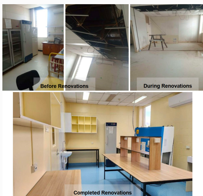
Figure 4: An example of a microbiology lab renovation
